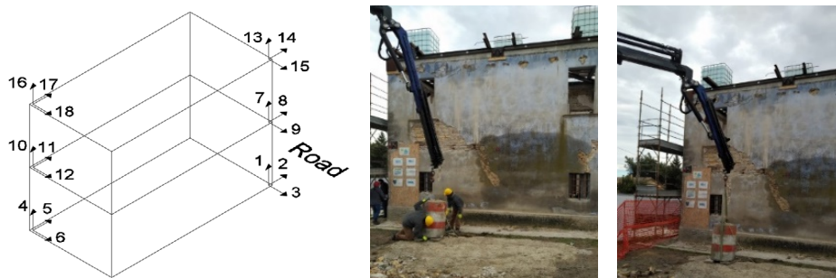
Fig. 5. Dynamic characterization: sensor deployment for each building and tests with mass drop.
